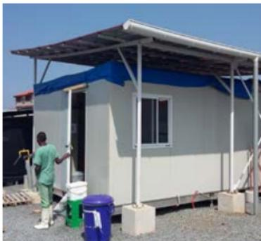
**M**SF's innovative laboratory consisted of an airtight metal shipping container spanning the High-Risk Zone (for patients and staff) and Low-Risk Zone (for services like the pharmacy). The container had a plexiglass partition between the zones and could be safely accessed from both sides.
